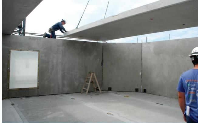
FIGURA 8. MONTAGEM DA LAJE PRÉ-FABRICADA (VISTA INTERNA)
